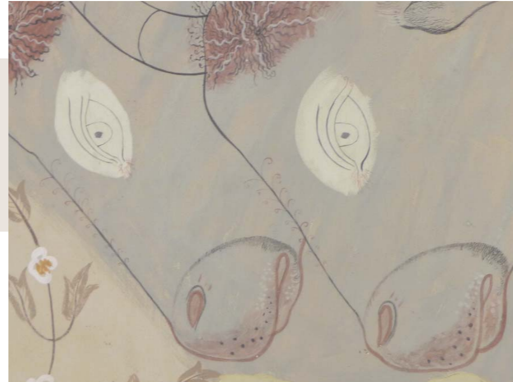
Detail of painted ceiling in what was originally the Small Refectory, Senate House.
